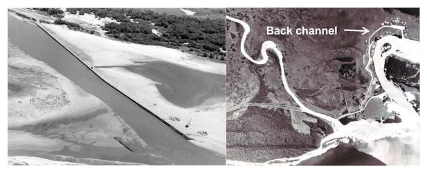
Figure 4.16. Armouring of the lower St Lucia estuary banks with cement-sand bags and dolosse (left, 1976) and the back channel excavated in 1970-71 (aerial photo from 1976) (Source: Illenberger & Clark 2014).
